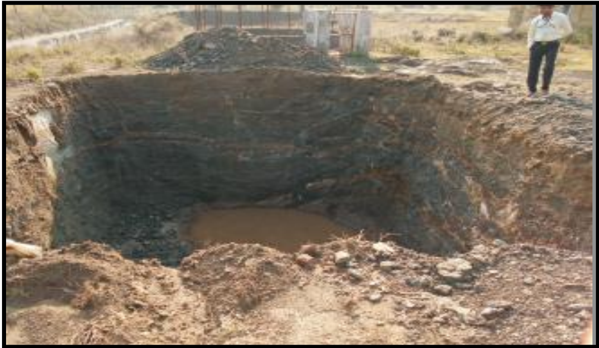
RAIN WATER COLLECTION PIT NEAR THE WELL.
